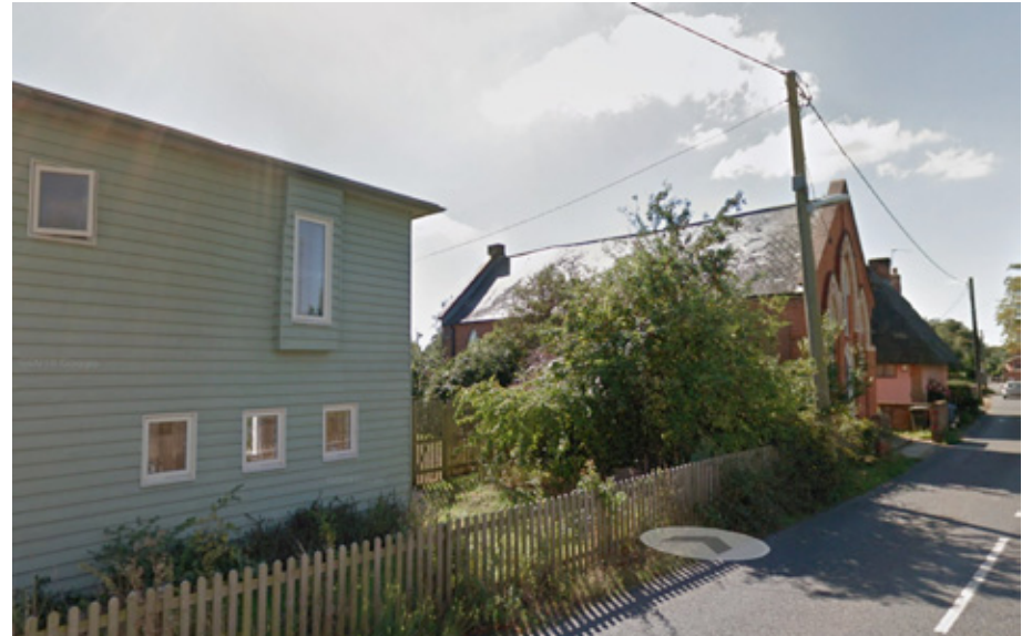
A mix of architectural styles along the village edge on Manningtree Road
